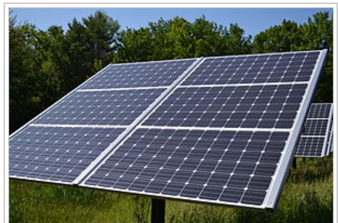
Fixed tilt solar array in of crystalline silicon panels in Canterbury, New Hampshire, United States
