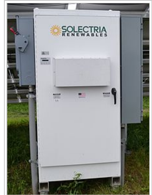
Central inverter with AC and DC disconnects (on the side), monitoring gateway, transformer isolation and interactive LCD.
