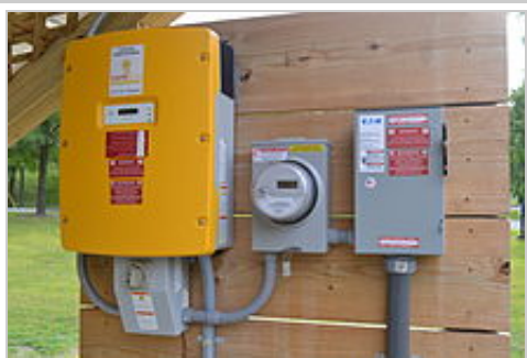
String inverter (left), generation meter, and AC disconnect (right). A modern 2013 installation in Vermont, United States.
