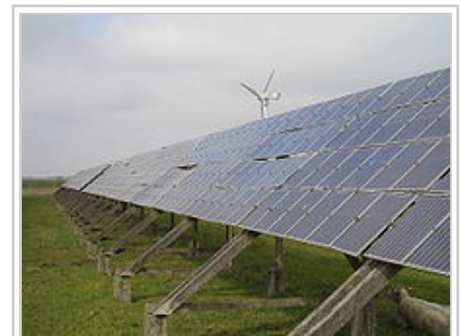
A 23-year-old, ground mounted PV system from the 1980s on a North Frisian Island, Germany. The modules conversion efficiency was only 12%.
